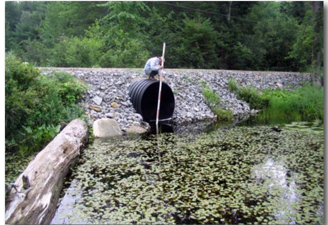
Measuring culverts as part of the Sheepscoot Barrier Survey.
